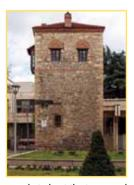
the so called teferiches. Two fireboxes were made to heat the tower and they were located in the walls on the first and second floor. The third floor was heated using the chimneys that passed through it. The stairs leading through the tower are placed in thick stone walls whose width is 1.45m.
