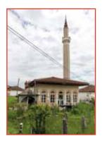
The slim minaret, located on the southwest side of the mosque and set on a square pedestal, dominates with its height and underlines the vertical emphasis of the mosque. The minaret body is polygonal and passes into the serefe through stalactite decoration. Although having modest architectural and decorative elements, the mosque reflects the local architecture in the second half of the 15th century dominated by clean and precise shapes.
